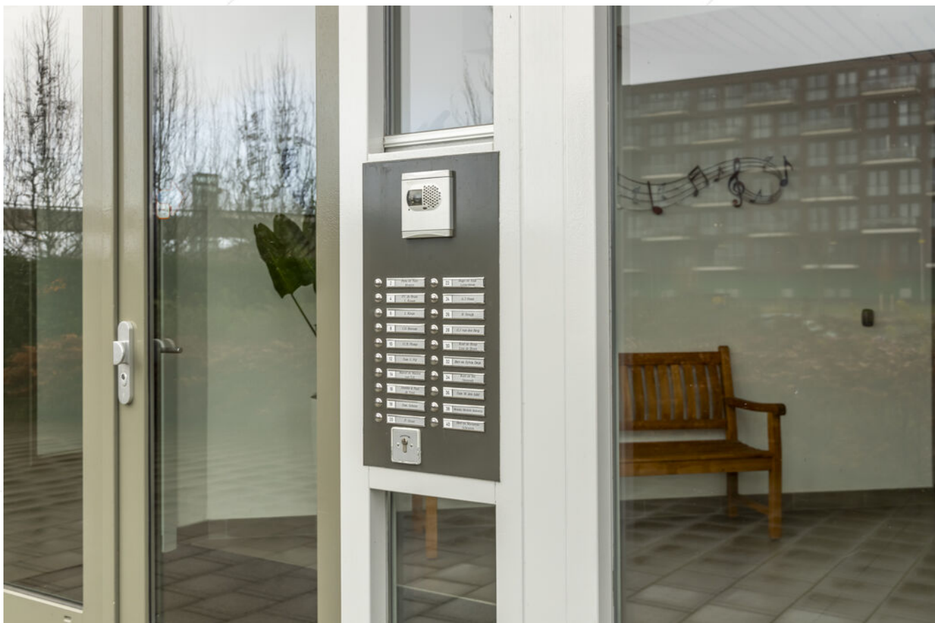
Centrale entree complex
