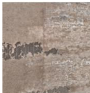
Contamination of condensers
