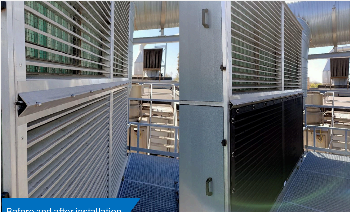
Before and after installation
